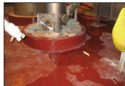
ARC NVE VC in service.
