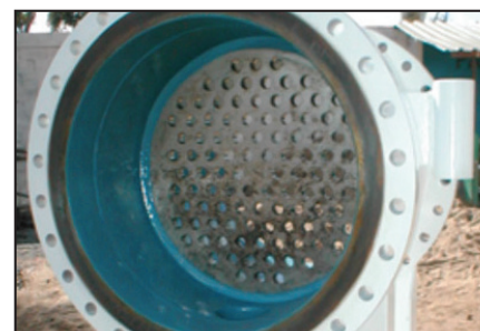
After cleaning and decontamination, ARC 858 is applied to fill and smooth surface.
