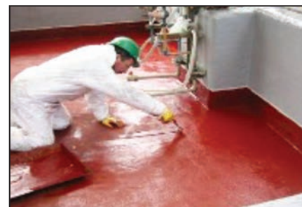
Applying ARC CS4 topcoat.
