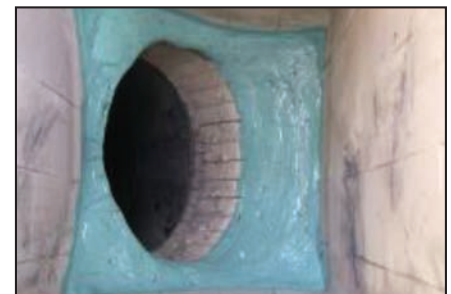
ARC BX5 with ARC S2 topcoat cures rapidly, allowing fast return to service of chute.
