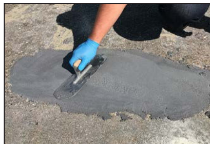
ARC EG-1 applied to concrete.
