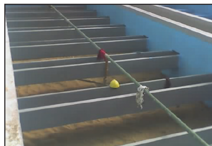
Installing ARC S1PW coating.
