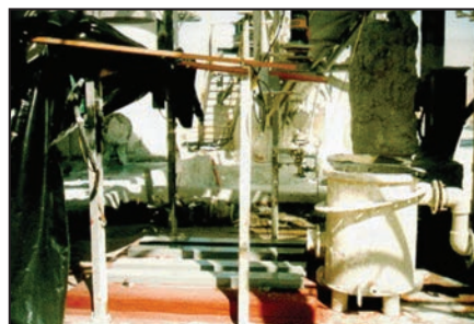
ARC 988 coated processing areas.
