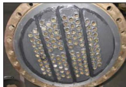
Completed tube sheet.
