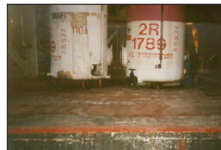
ARC 988 coated floor areas.
