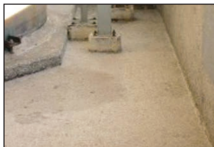
Cleaned and prepared surface.
