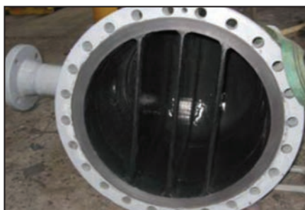
Repaired divider plates.
