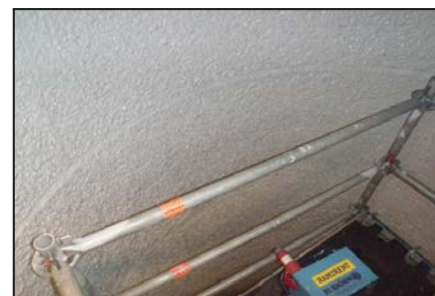
Surface of wet well with final coat of ARC S1HB.
