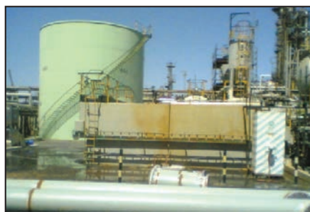
Basin in petrochemical complex.
