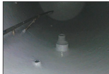
Coated tank internals.
